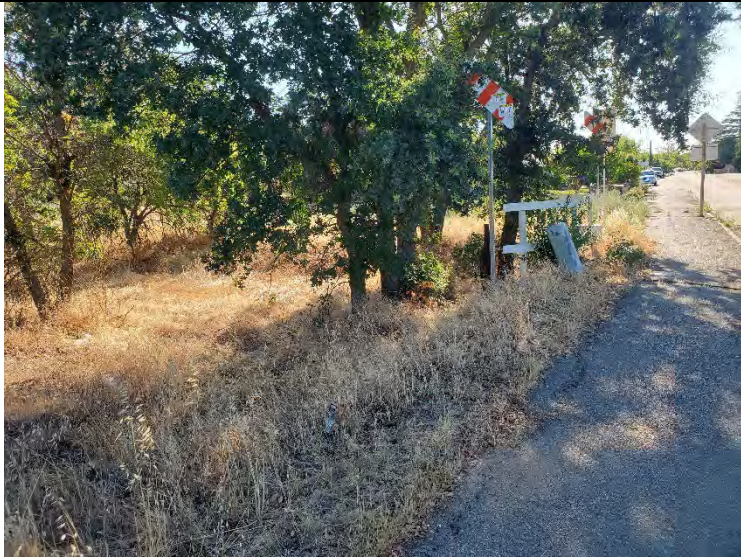
Facing east towards culvert along Main Street.
